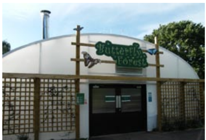
The Butterfly House, with boiler fitted.
